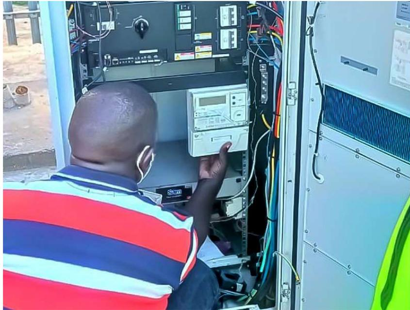
Installation of AC and DC controllers equipment is carried out WITHOUT DISCONNECTING consumers and interrupting the operation of the BS.
